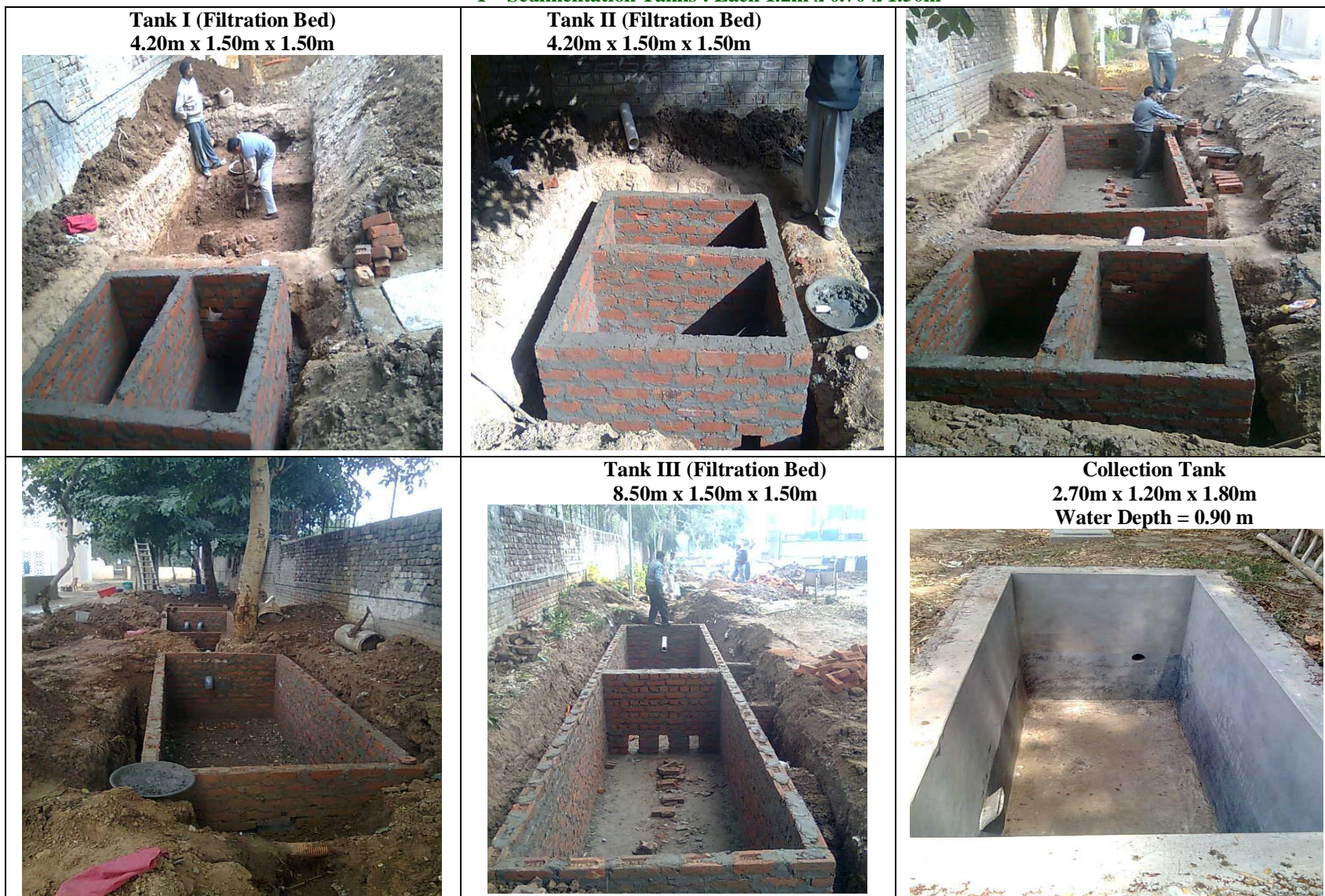
Fig. 2: Constructed wetland: A Pilot Project to treat Institute Hostel Mess wastewater I – Sedimentation Tanks : Each 1.2m x 0.70 x 1.50m
