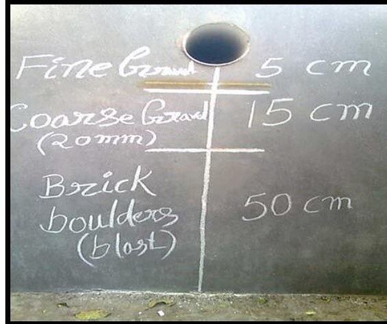
Fig. 3: Constructed wetland: Hostel Mess wastewater treatment and filtration beds.
